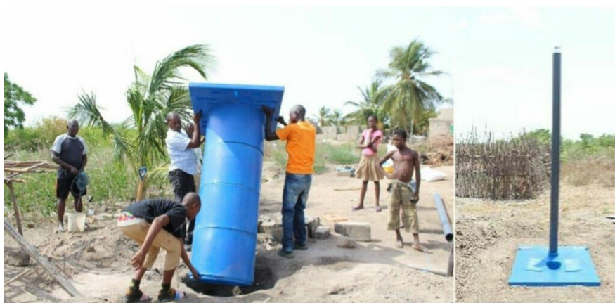
Figure 9: Digni-Loo installation in Ghana, showing the full lining (left) and the final installed product (right) (source: Global Communities Ghana)
