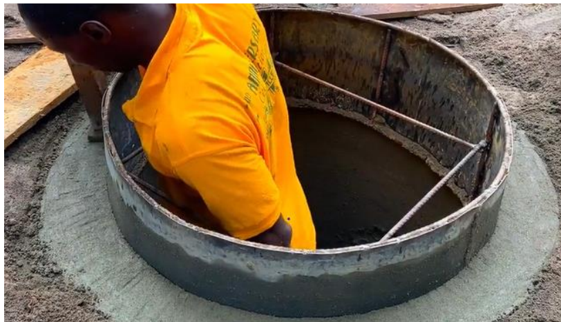
Figure 5: Construction of cement-reinforced stabilized soil lining (source: CAWST)
