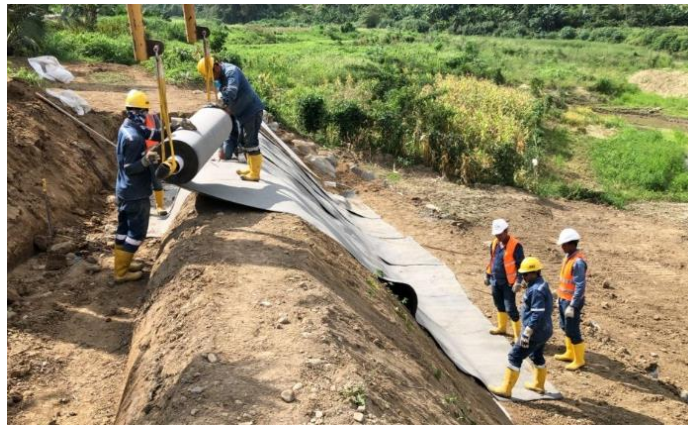
Figure 7: Rolling out concrete canvas during construction (Source: Geosynthetics Magazine)
