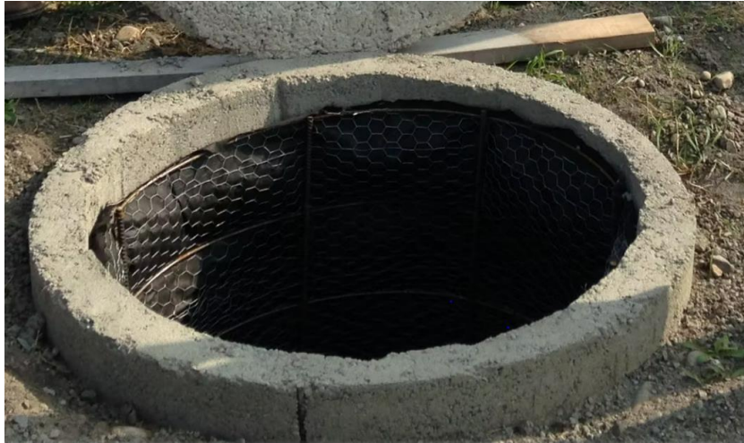
Figure 4: Rebar-reinforced fabric lining (source: CAWST)
