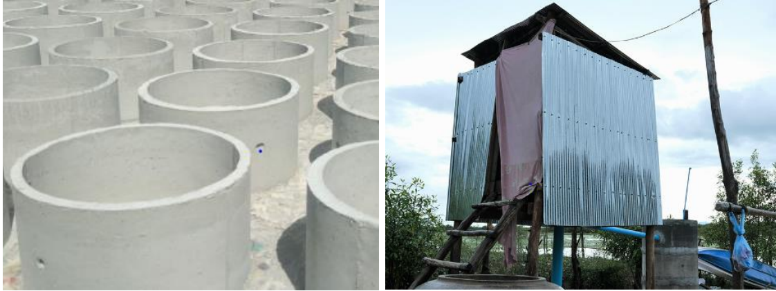
Figure 3: Wet Ring for iDE's Easy Latrines in Cambodia (left, source: iDE Cambodia), used for Sky Latrines constructed on stilts for seasonally flooded areas (right, source: Water For Women Fund)
