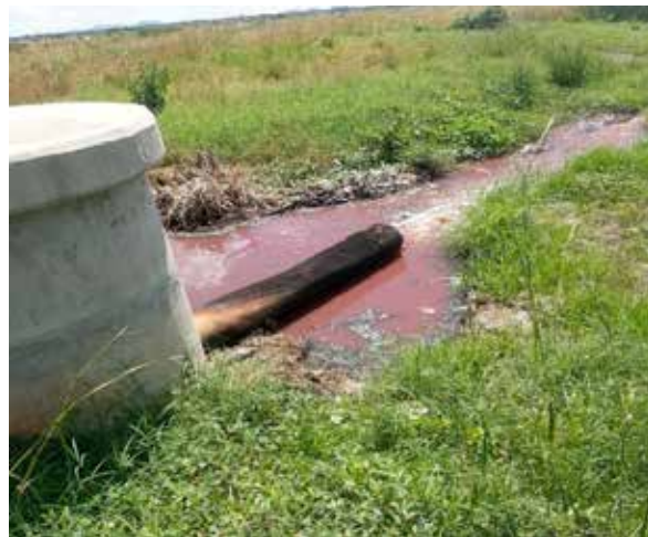
Figure 3.7: Red Effluent at the outflow of Roton Wastewater Lagoon
