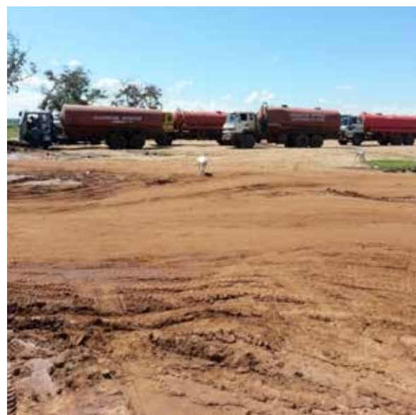
Figure 3.4: Unpaved and poorly maintained Access Road to Roton Lagoon
