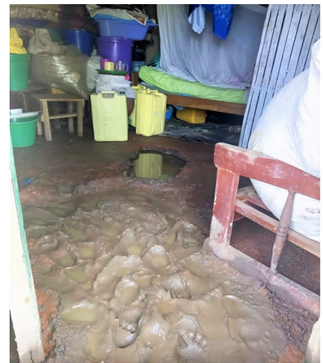
Photo 7: A house in Paicho sub county flooded because of high water table problem in the area.
