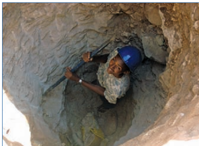
USAID funded the construction of this hand-dug well in Ethiopia's Somali region
